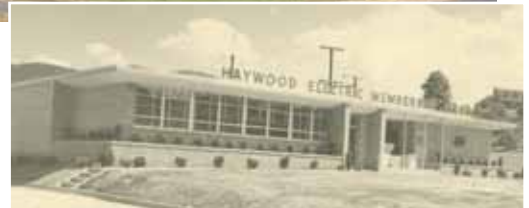
Top: Haywood EMC's new office facilities in Waynesville. Inset: The co-op's original office facility built in 1953.
